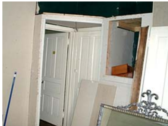
Original entrance to bedroom and wall against steps.
