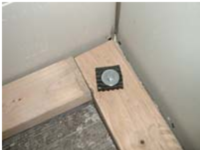
Inner framing with Vib-X washer.
